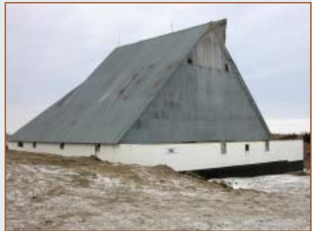
Sands Barn Roof on new foundation, February 9, 2007.
