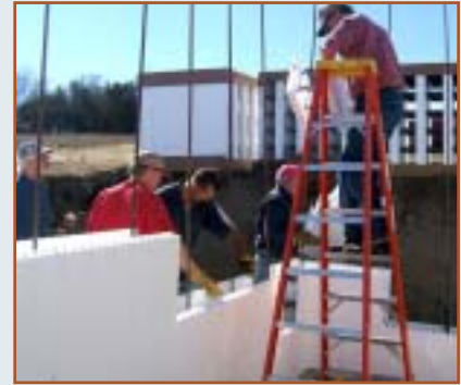
Volunteers assembling insulated concrete forms and framing.
