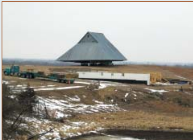
Semi tractor ready to turn the barn roof around on the prairie hill overlooking the Platte River Valley.
